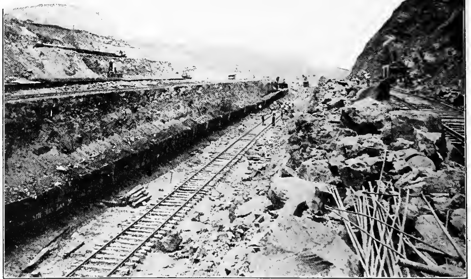
CUTTING AT BASE OF CONTRACTORS HILL
